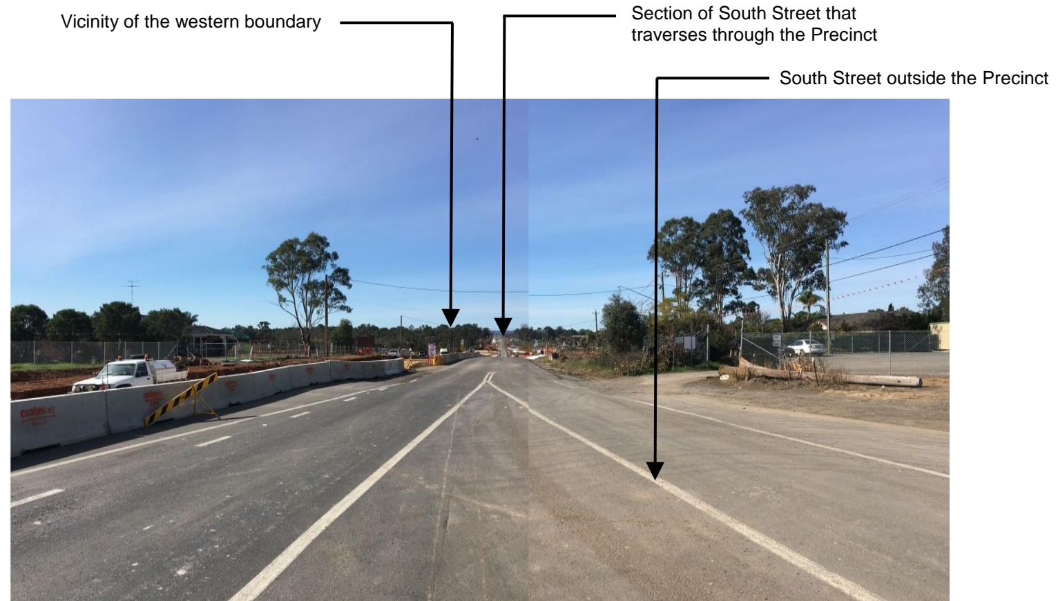
Site Context Photograph 5: View looking east towards the Precinct from South Street
